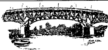
Granville Street Bridge, Vancouver, BC
