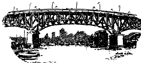
The Granville Street Bridge, Vancouver, BC
